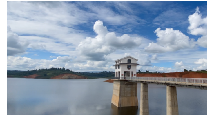
The Karimenu II Dam Water Supply Project will provide 70,000 cubic meters of clean drinking water every day for capital city Nairobi
